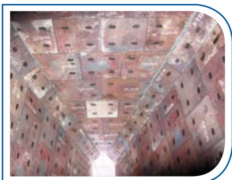
Typical chute with liners bolted into place
