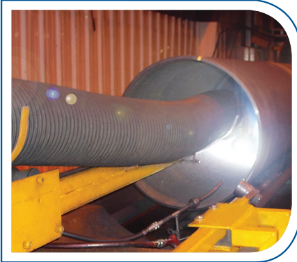
Pipe overlay machinery - the most advanced and efficient in North America
